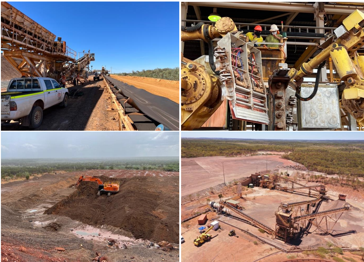
Images 3-6. Stacker refurbishment, robot calibration, crushing circuit maintenance, heap leach re-working.
