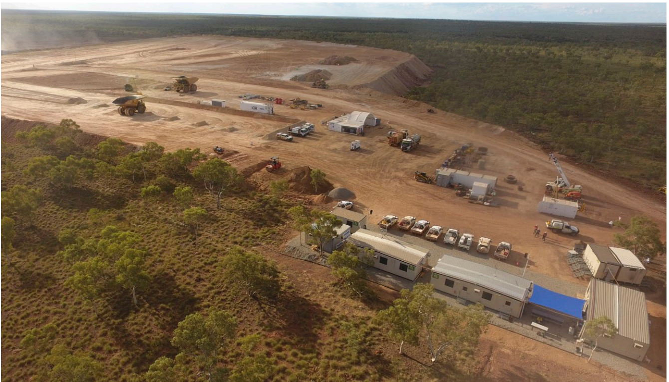
Anthill Mine site offices.
