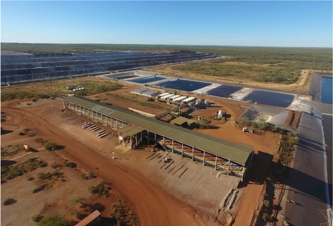
Mt Kelly processing plant; electrowinning tank house in the foreground, solvent extraction circuit in centre, and heap leach in background.
