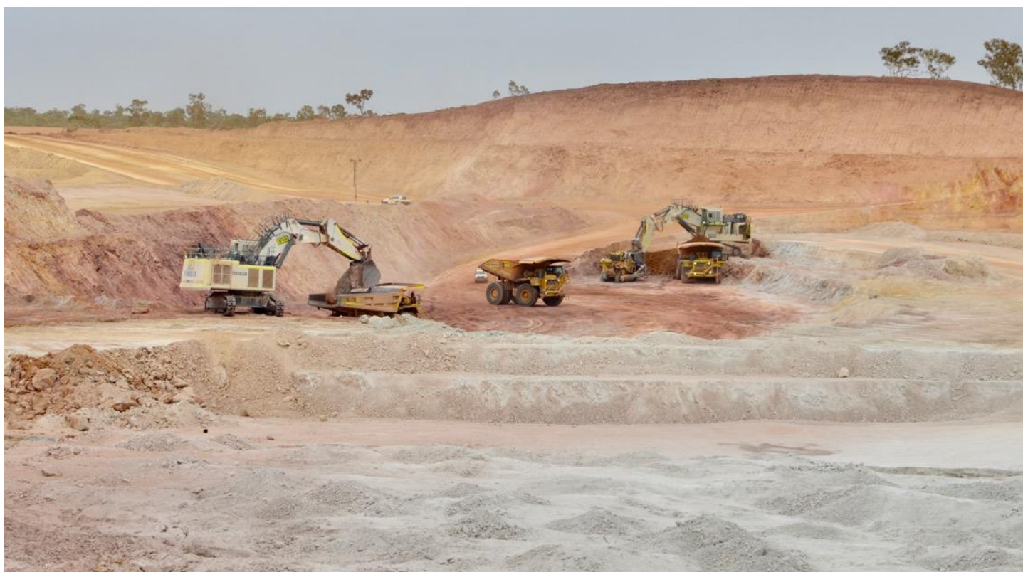
Figure 10. Anthill Mine east pit 23 April. Both excavators are mining ore.
