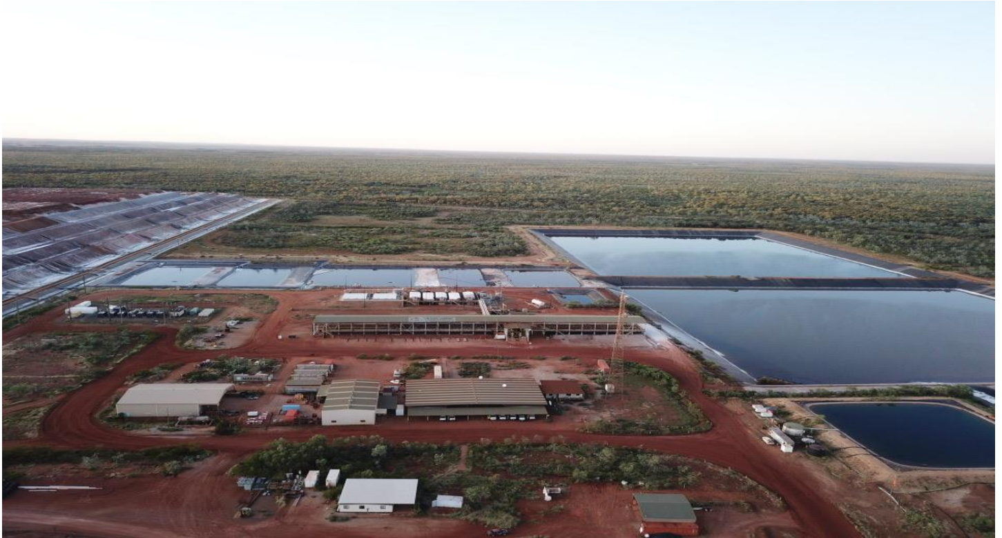
Figure 8. Lady Annie Processing Facility looking South.
