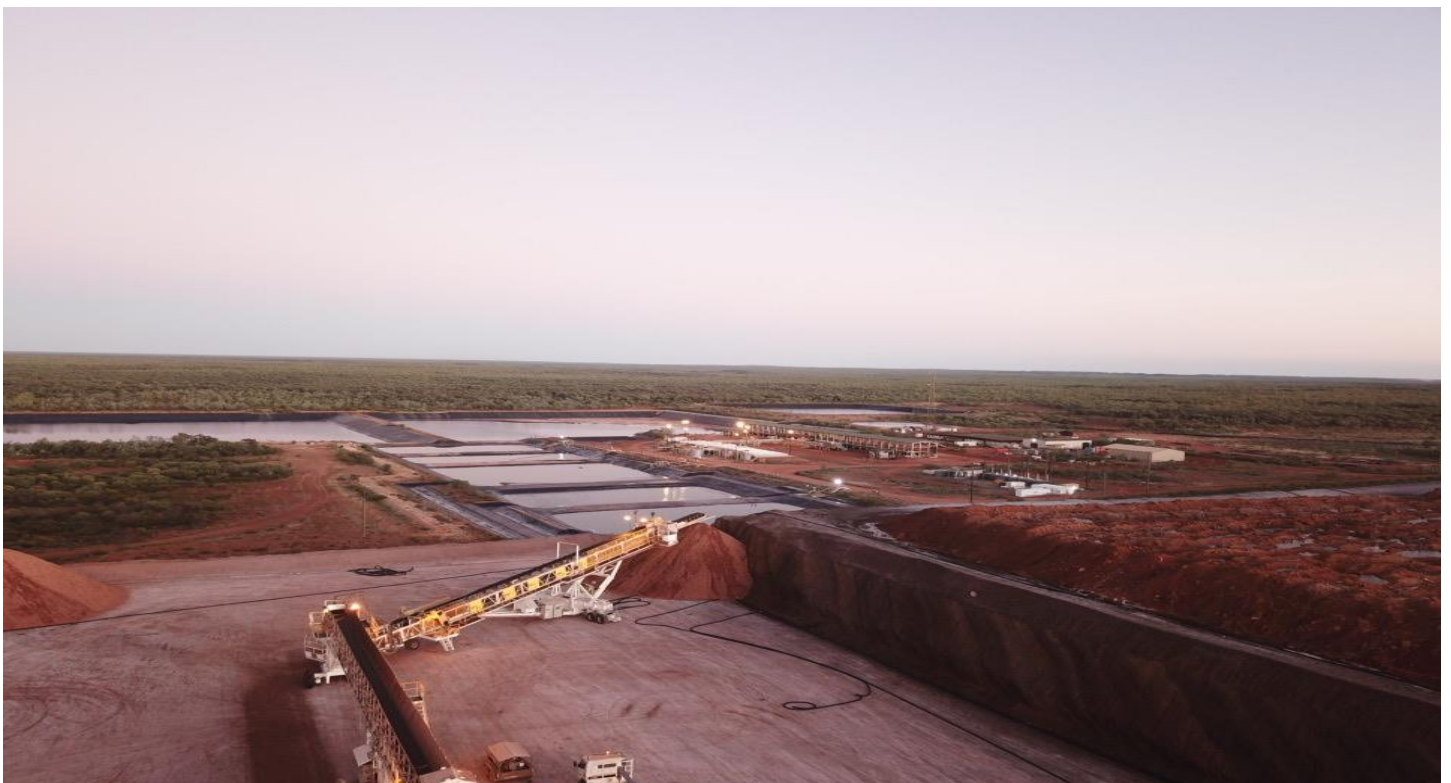
Figure 9. Stacking ore on the Heap Leach Pads.
